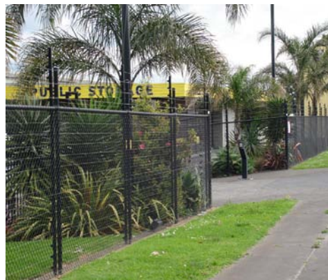
Electric fencing can be added to existing fences
