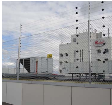
8 foot electric fence installed on existing wall
